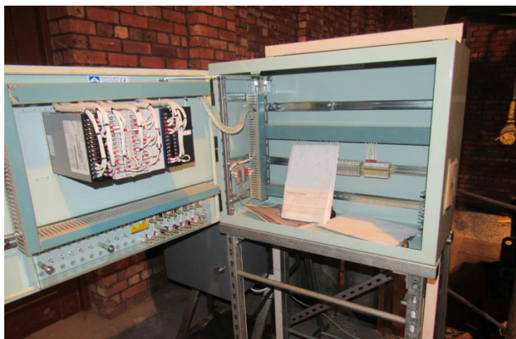
Figure 2.7: Internal view of the FCL service protection (AP panel)
