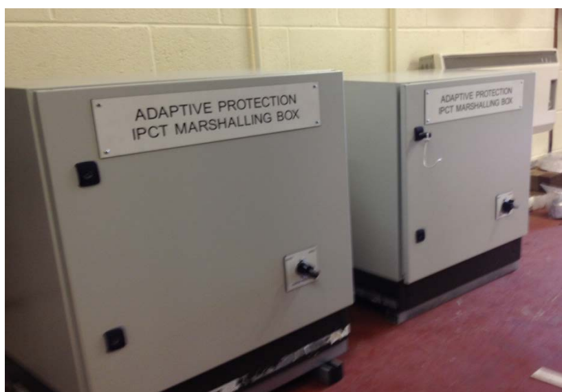
Figure 2.2: Interposing CTs removed for the simplified installation at Denton West
