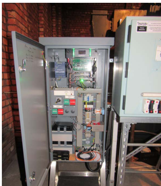
Figure 2.7: Internal view of the FCL service protection (AP panel)
