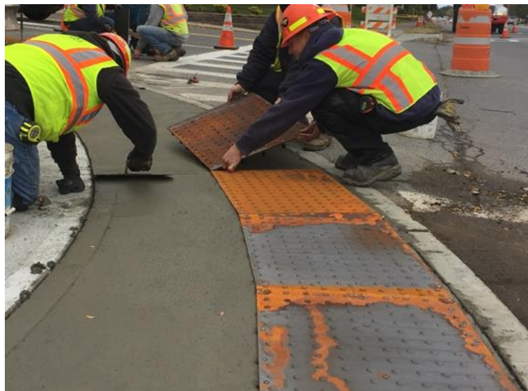
Figure 6 The front edge of detectable warnings placed at the back of curb cannot be more than 2 in. from the back of the curb. Rectilinear units used on a radius typically need to be cut to maintain a compliant, continuous detectable warning surface along the entire the width of the pedestrian access route.
