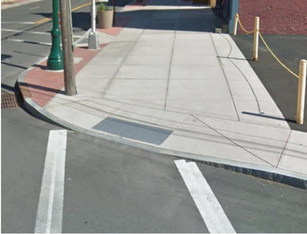
Figure 7 The domes of detectable warnings should be oriented perpendicular to the lower grade break of a ramp. They do not need to be oriented to the pedestrian crossing. Both of these installations are correct.
