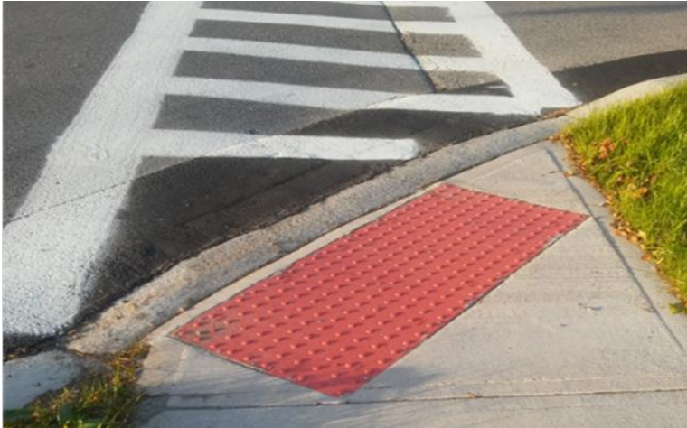
Figure 3 This detectable warning installation is incorrect: the surface does not cover entire width of the accessible route.
