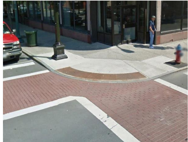
Figure 7 The domes of detectable warnings should be oriented perpendicular to the lower grade break of a ramp. They do not need to be oriented to the pedestrian crossing. Both of these installations are correct.
